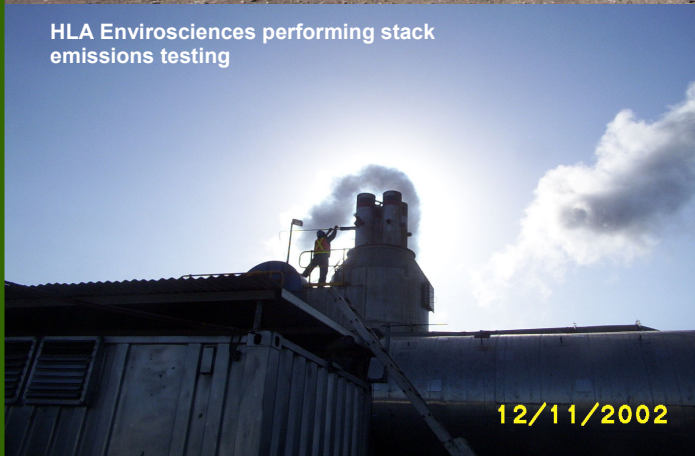
DFTD process in operation on the BHP site, Newcastle
