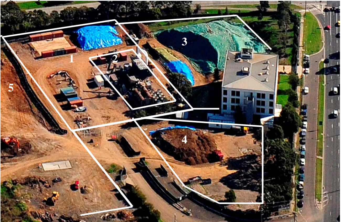
Figure 3 – The Thermal Desorption Treatment Layout at Springvale
